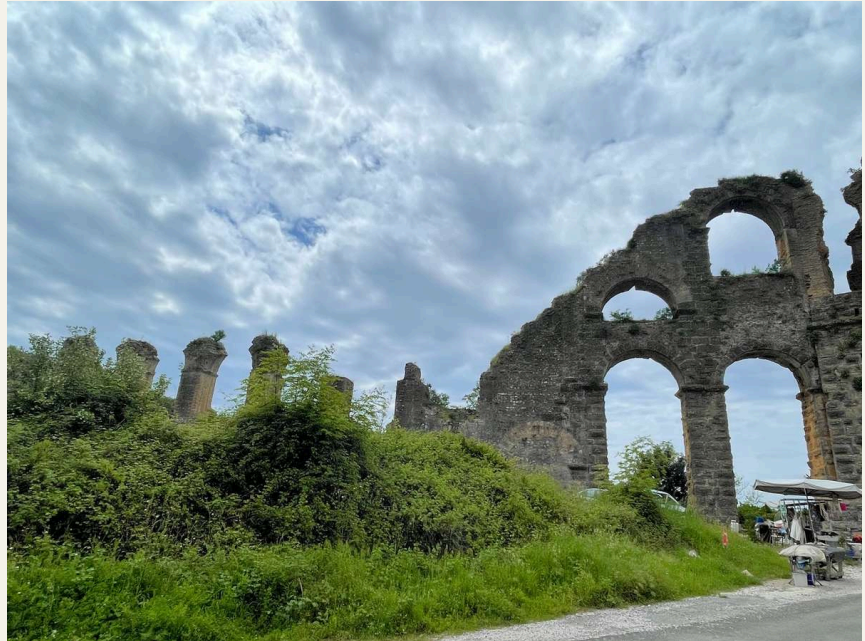
The aqueduct at Aspendos
